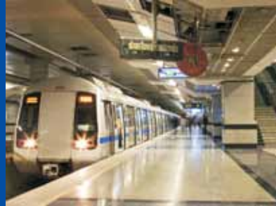
Barakhamba Metro Rail Station, New Delhi Construction by AFCONS
